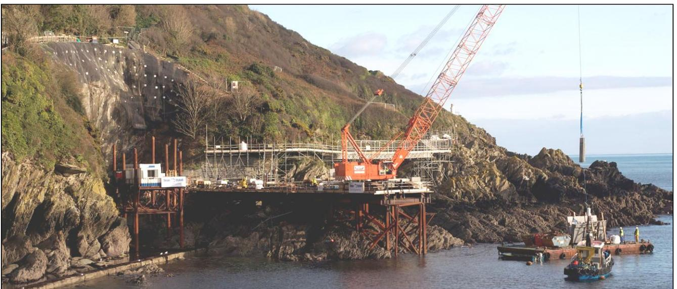
*Equipment and pre-cast concrete units (for the Screening Building) being delivered by sea barge to Scilly Cove from Par Docks*
