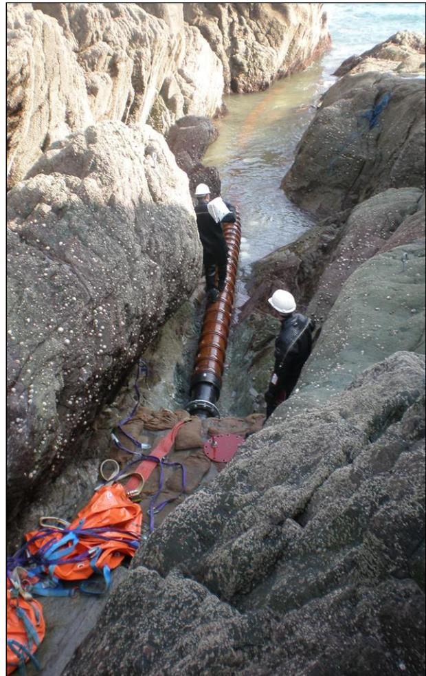
*The new intermediate section of the gully outfall pipeline was installed during calm sea conditions*
