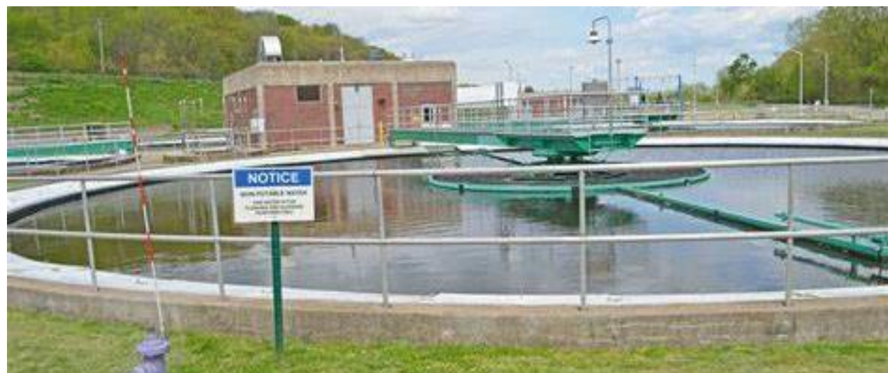
Sewage Treatment Works Upgrade
