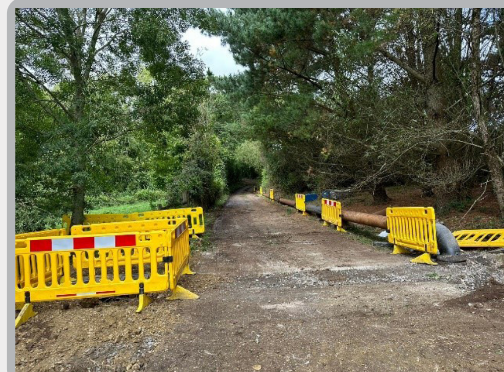
The temporary overland solution used for the Uplyme Rising Main
