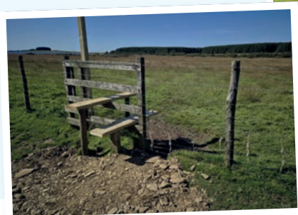
Below Stile repaired and stone placed, Crowdy Marsh
