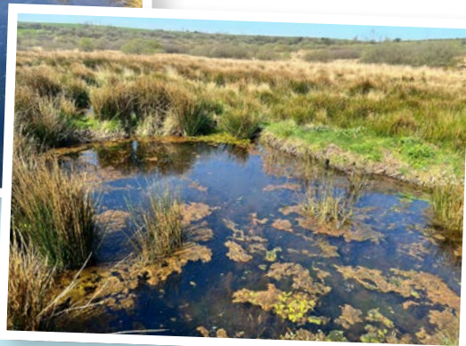
Peatland restoration at Park Lake
