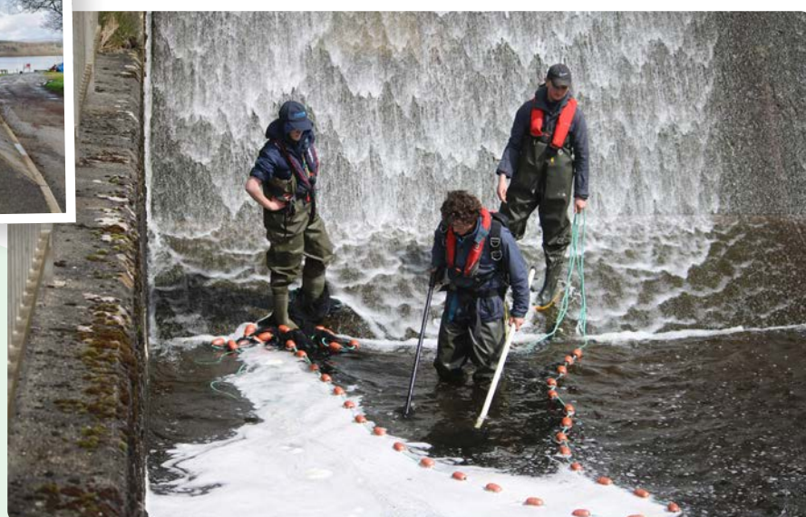
Above left Wash down facility at Roadford Lake
